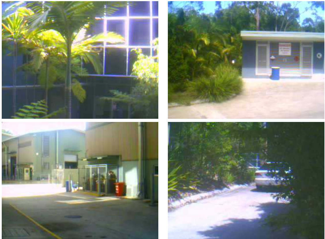
Figure 6.1: Sample images taken by the wireless sensor network camera system.
